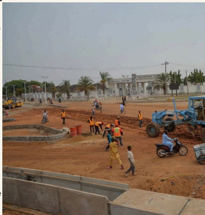
Road reconstruction in Gusau, with Government House visible in the background.
